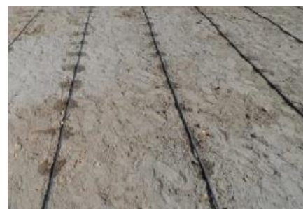
Fig.6 Lateral pipelines for dripping
